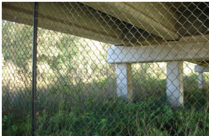
Along the SunCoast Parkway in Pasco and Hernando Counties, bridges were designed with well vegetated underpasses and high fencing to discourage wildlife from venturing up onto the highway.
