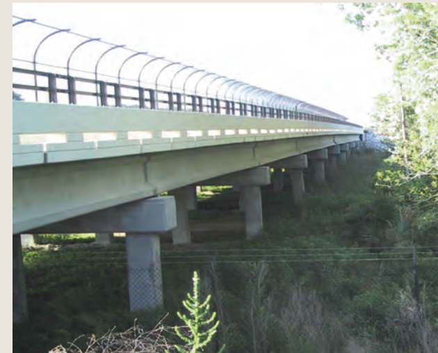
Photo showing bridges constructed to allow for good vegetative coverage and wildlife connections.
