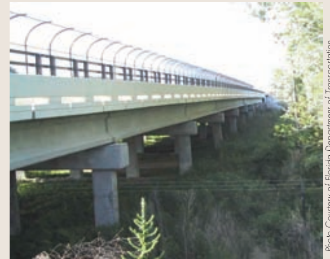
Photo showing bridges constructed to allow for good vegetative coverage and wildlife connections.
