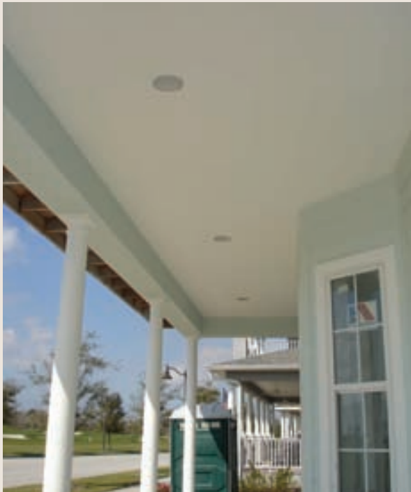
Outdoor lighting can be designed to lessen light pillage into the surrounding night sky.
